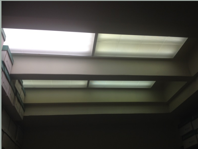
Shallow surface-mounted 2'x4's – before and after custom kit
